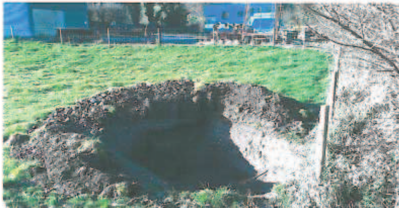
Hole dug in field (by others) opposite Farmcomb Farm – note water in base
