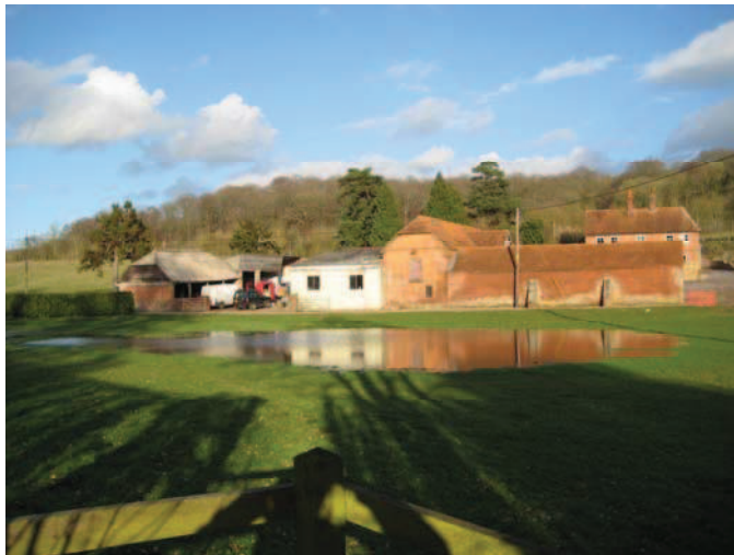
Figure 4: Surface water flooding at Whitfield Farm (200mm)
