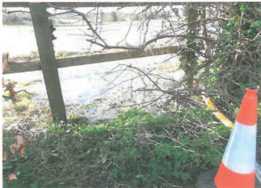
LAM013. Windsor House Paddock. 15 FEB. 2014 View from Crowle Road, showing extent of water across horse track/gallop. Pump carrying water into drain, marked by cone.
