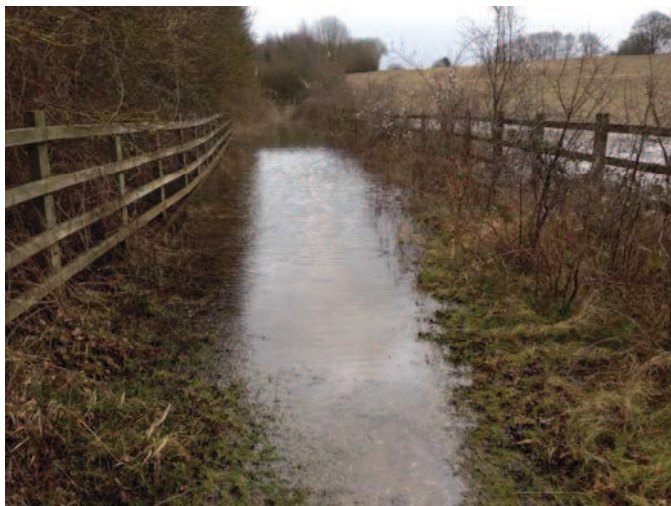
Figure 6: Flooding at public footpath west of A339 near Vodafone (300mm)
